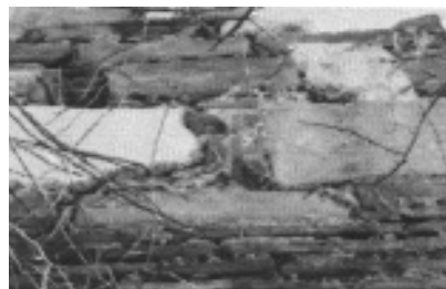
Figure 22. The brick decoration in “e” section tower II
