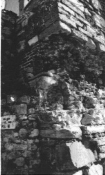
Figure 23. The traces of brick courses in “j” and “k” sections tower III
