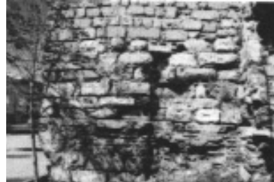
Figure 19. The “c” section in west defence line
