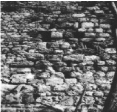
Figure 24. The cavities in “i” section tower II
