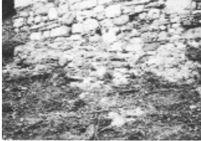
Figure 14. The mortar stone constitutes the footing of garden wall
