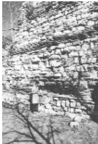
Figure 17. The traces of west defence line upper section
