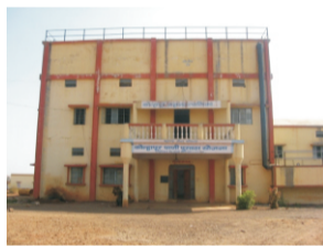
Plate-1 Puikhadee WTP located at 14 km from the city on Kolhapur- Radhanagari road.
