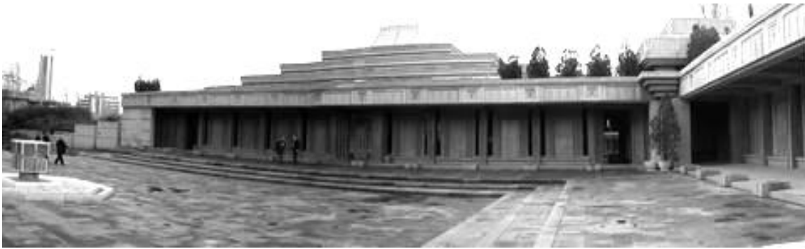
Figure 6. North Facade, TBMM Mosque (Photograph by Özgür Ürey)
