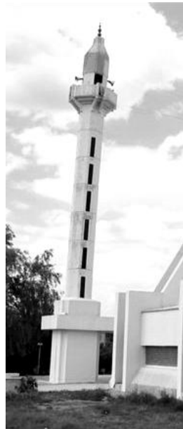
Figure 5. Minaret, TEK Mosque (Photograph by Özgür Ürey)
