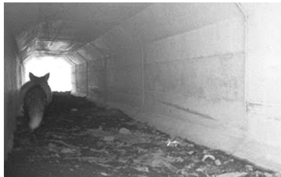
Figure 4. Medium size underpass (URL-1)
