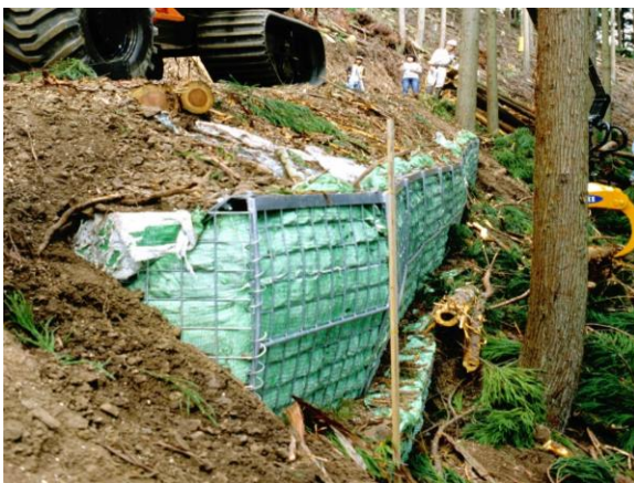
Figure 2. Retaining wall (L-shaped steel retaining wall) utilizing road width efficiently
