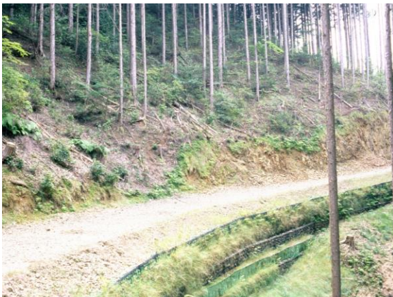
Figure 1. Retaining wall (L-shaped steel retaining wall) crossing crushing zone
