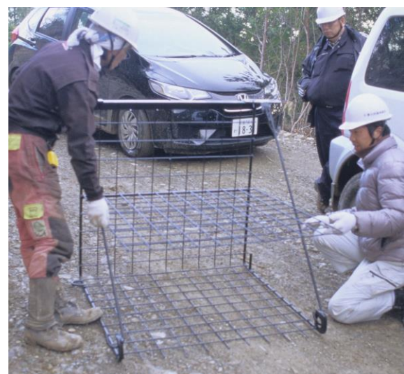
Figure 3. Structure of L-shaped mesh wall
