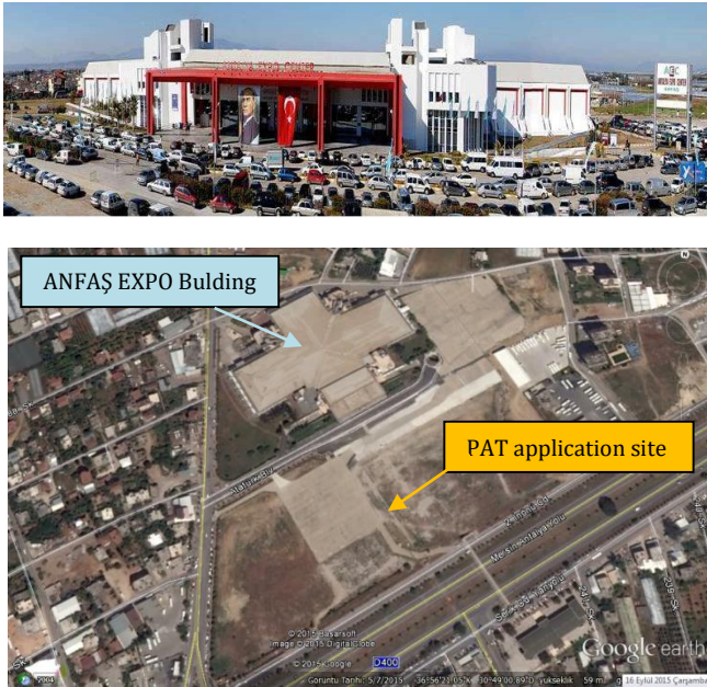
Figure 10. Antalya ANFAŞ-EXPO building and location of PAT application site
