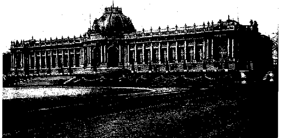
Figure 3. The second project for the residence in Leopoldville, by architect M. Vander Elst 1925 (Africa Archives, Brussels).
