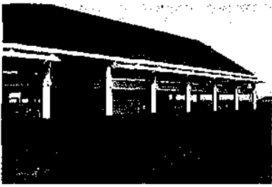
Figure 3. Part of new campus designed by Summet Jumsai for Thammasat University near Bangkok, Thailand. Jumsai's regionalism is inspired by South East Asian "houses-on-stilts" as well as planning principles of the "temple city" of Angkor Thom, Cambodia. The design responds to both the local climate and landscape as well as the functional needs of a modern university (photograph by author)
