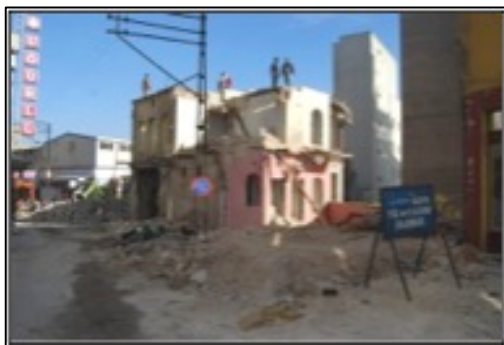
Figure 24: Street Widening Works
