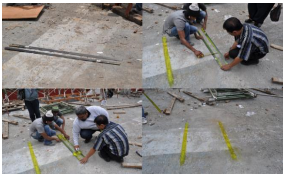
Figure 19. Implementation of Measurement and concrete surface markings
