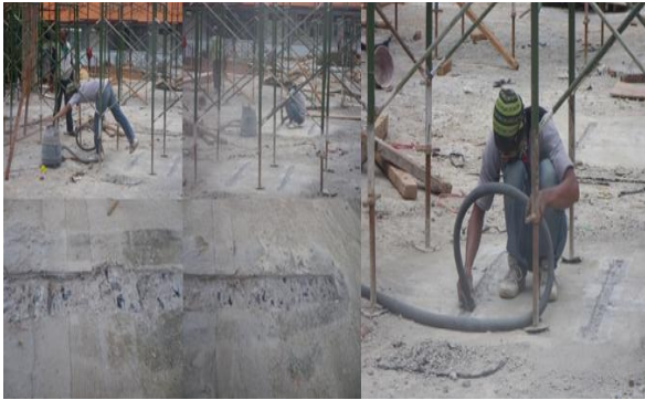
Figure 18. Implementation process and results Patching
