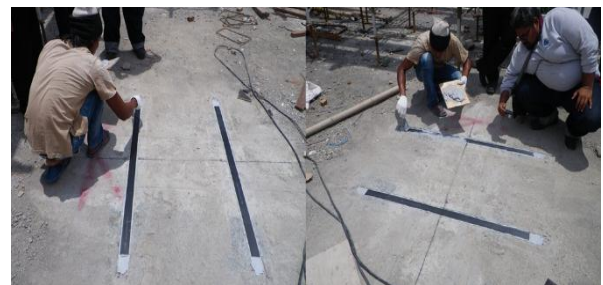
Figure 20. CFRP installation process
