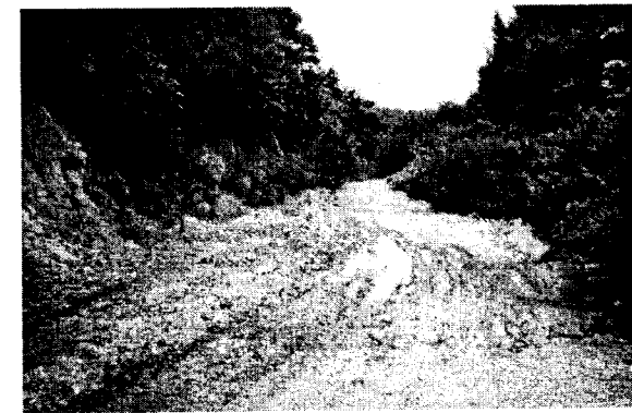
Figure 3. The conditions of 02 code forest road, ditch, and roadbed prior to pavement activities (Photo: T.Ozturk)
