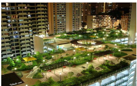
Intensive green roof
