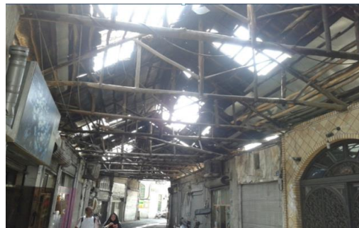
Figure 17. Marketplace's roof after the restoration (source: cultural heritage)
