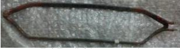
Fig.3. The coil of 6kv generator tested
