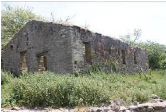
Fig.17: Bademliköy, zeytinyağı imalathanesi.
