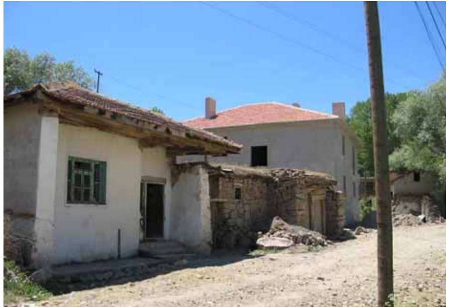
Figure 5. One type of hybrid existence is the saved older mudbrick or stone structure sitting next to a new, oversized, free standing, in-filled concrete frame structure (A. Snyder, 2002).
